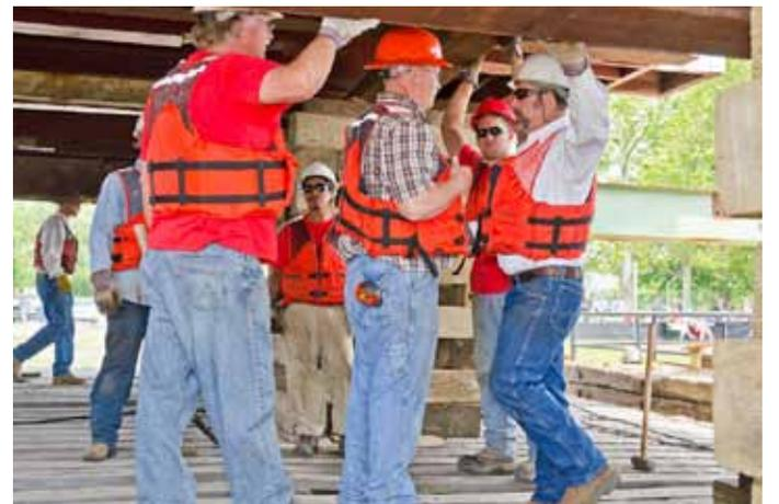
It was originally thought that the Roanoke River Lighthouse could remain at land; however complications arose and it was decided to put the lighthouse on pilings near the shore to show how it would have looked when it was out in Albermarle Sound. The lighthouse was moved to its new site on rollers that moved the structure about three feet at a time and was accomplished in less than a day's time.
